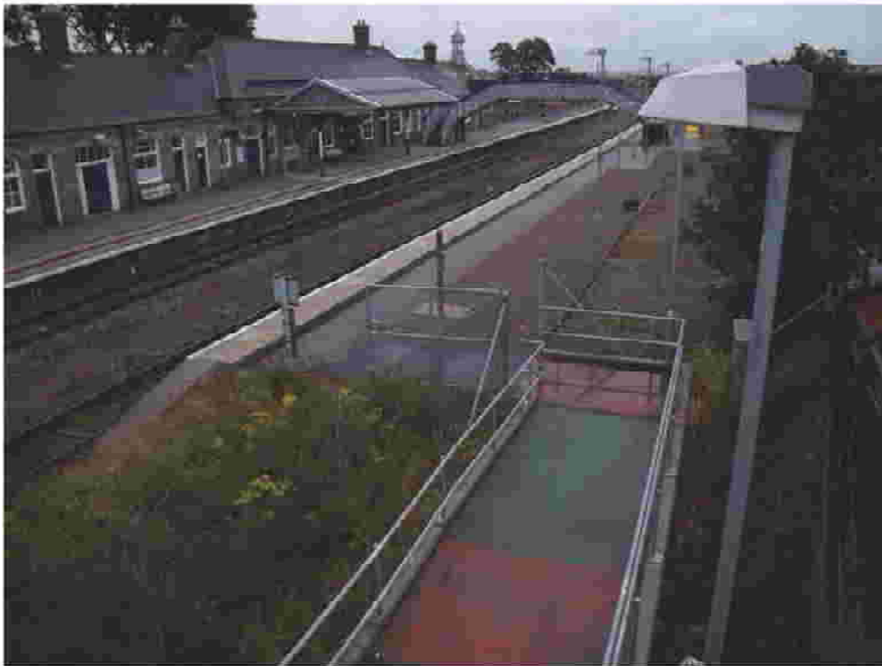
Graded ramp for wheelchair users at Inverurie Platform.
